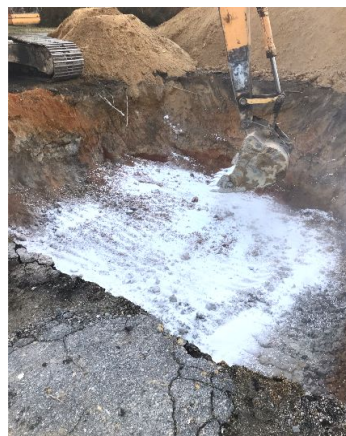
Figure 2. Excavation area below former dispenser island and the RemRx ™ CRP deployment.
