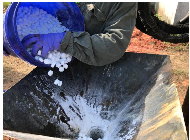
Figure 2. Backfilling of the hollow stem auger borings with RemRx TM CRP Persulfate pellets. Borings were loaded with persulfate (to overcome SOD), pellets, and persulfate activator.
