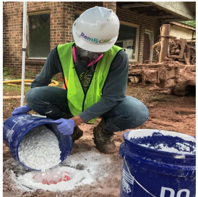
Figure 2. Backfilling of the borings with RemRx TM CRP Persulfate pellets. Borings were loaded with persulfate (to overcome SOD), pellets, and persulfate activator.
